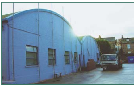
Before: Barrel Roof
