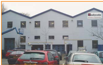
Before: Pitched Roof
